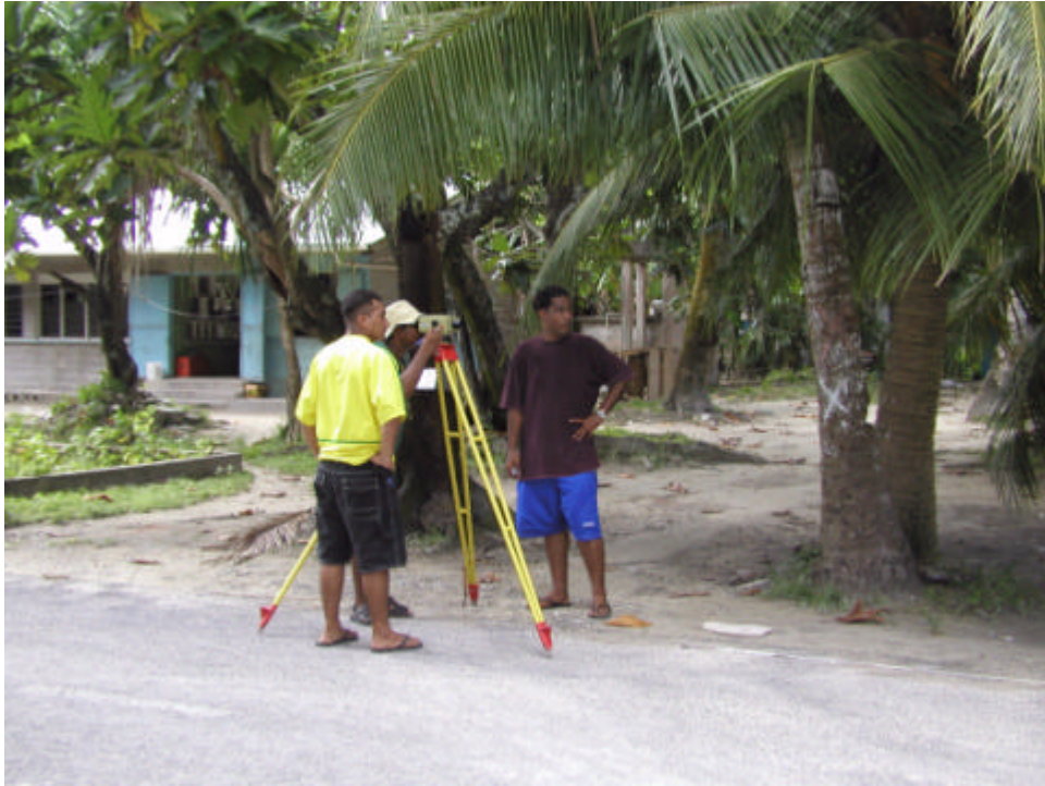
Levelling along main road
