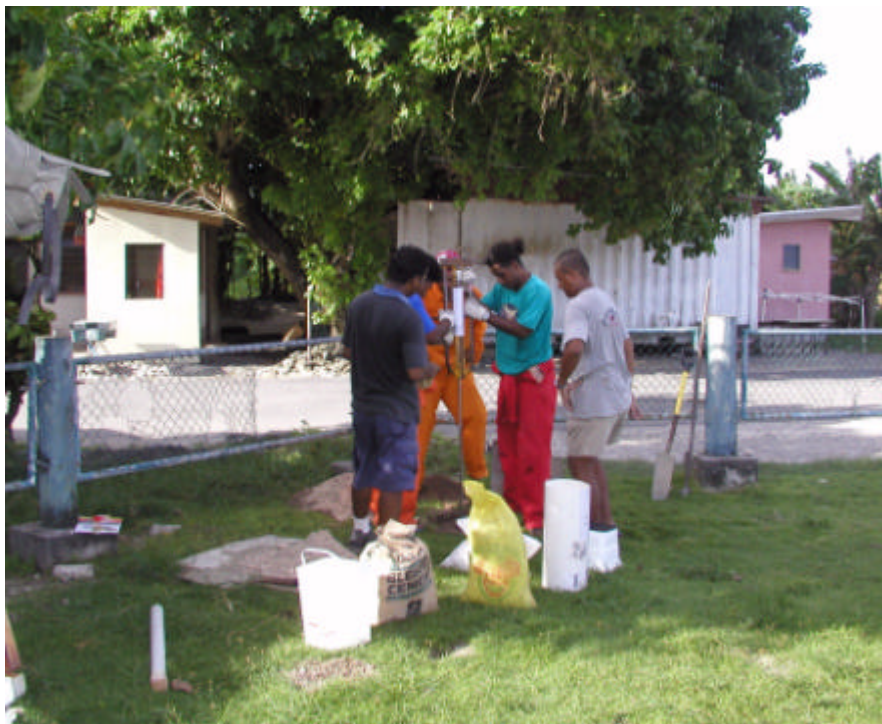
Installation of deep benchmark, BM 27
